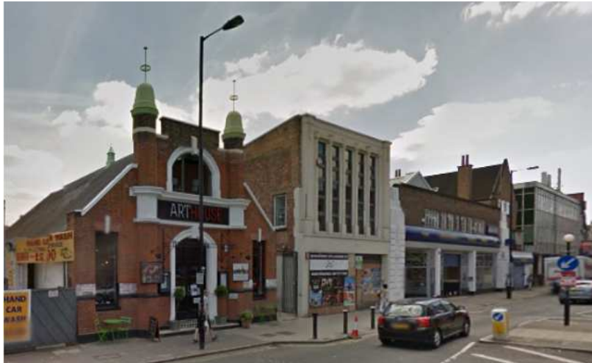
Photo 3: Existing front elevation with Art House Cinema to left and Kwik Fit garage to right
