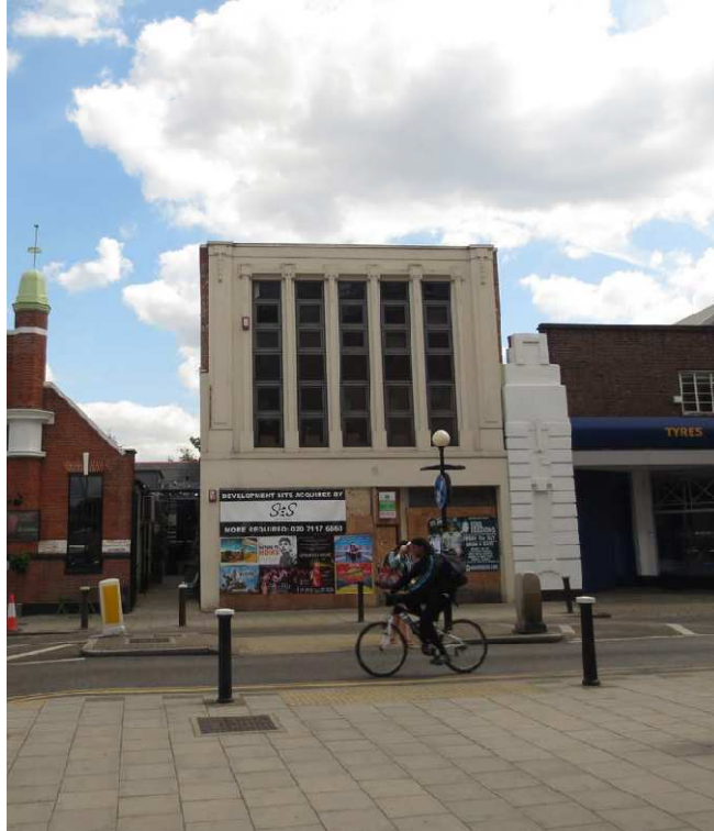
Photo 1: Existing front elevation
